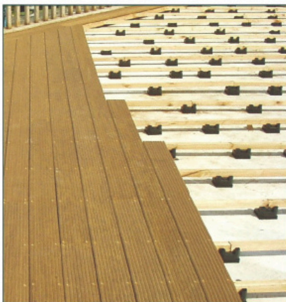
DECK DETAIL FOR ROOF DECKING WITH SHOCK ABSORBING LEVELLING CRADLE
